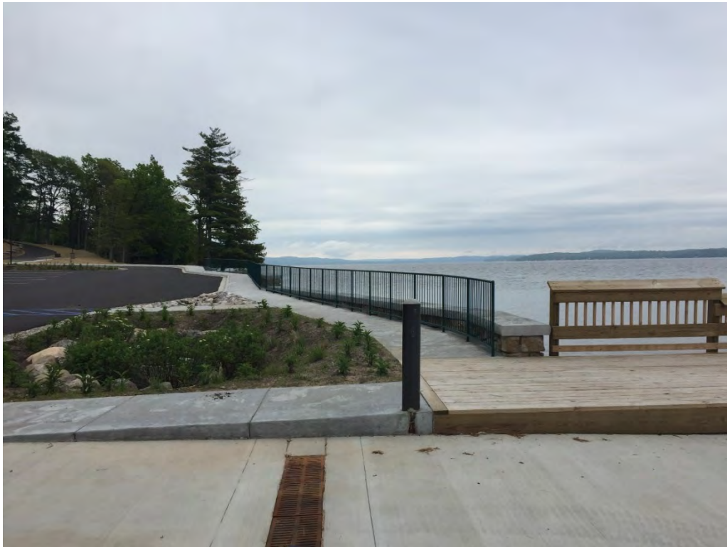
Photo # - Safety Rail Along Break Wall
