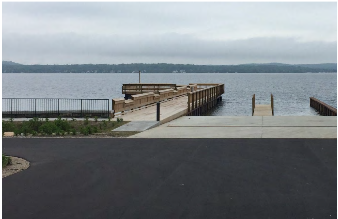
Photo # - Pier Guard Rail
