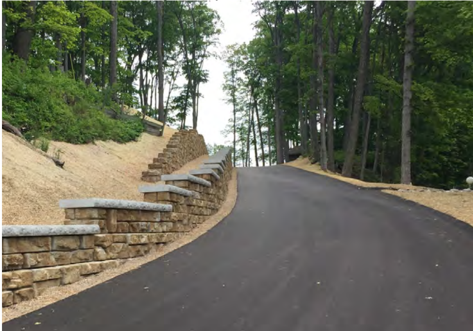
Photo # - Safety Railing Along the Turf Path Wall Structure
