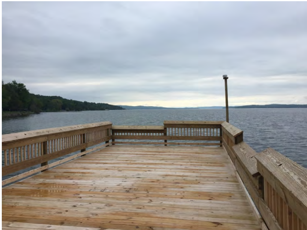
Photo # - Pier Guard Rail
